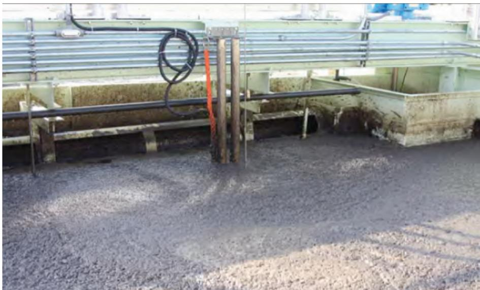
Figure 3. Foaming Observed at Sturbridge Wastewater Treatment Plant (from Catlow & Woodard, 2012)
